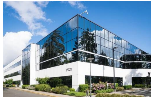
Facilities Maintenance (commercial)
